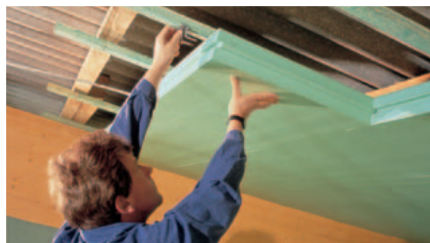
Fig. 7: Fixation of Styrodur C boards.
