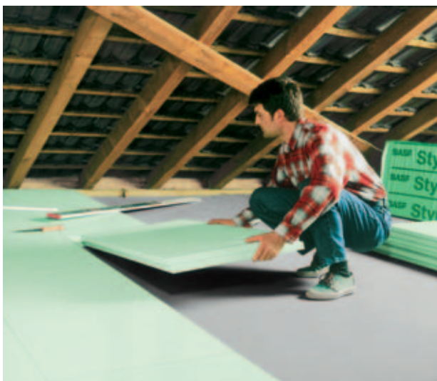
Fig. 4: Insulation of an attic with Styrodur® C.
