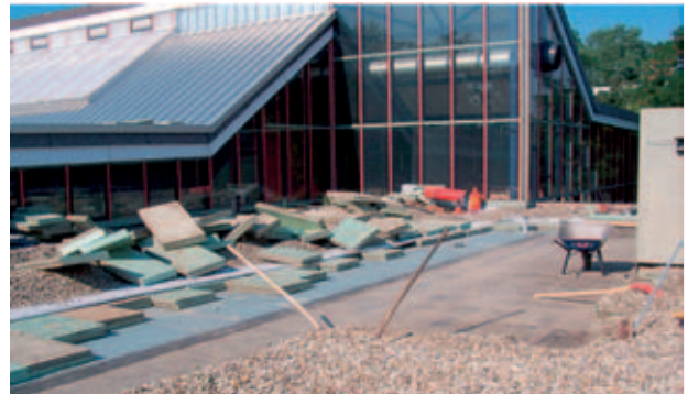
Fig. 1: Reconstruction with Styrodur® C.
