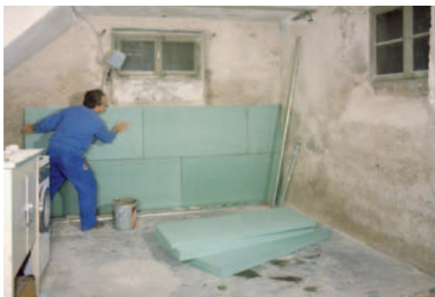
Fig. 27: Thanks to its properties, Styrodur® C is also suitable for the interior insulation of basements.
