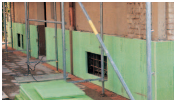
Fig. 19: Subsequent base insulation with Styrodur® 2800 C.
