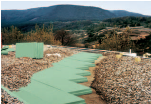
Fig. 6: Reconstructed inverted roof as plus roof construction.
