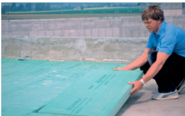
Fig. 4: Installation of Styrodur® C insulation on roof.
