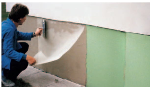
Fig. 20: Fiberglass grid is fixed onto the plaster.
