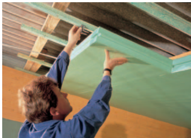
Fig. 12: Fixation of Styrodur C boards.
