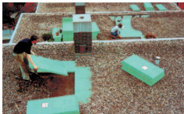
Fig. 5: Installation of thermal insulation under gravel.
