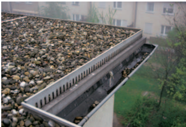
Fig. 7: Gravelled roof on Styrodur® C.
