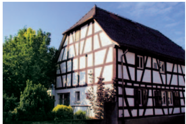
Fig. 2: Styrodur C is used for the reconstruction project of this old timber-frame house, organized in cooperation with dena (German Energy Agency).
